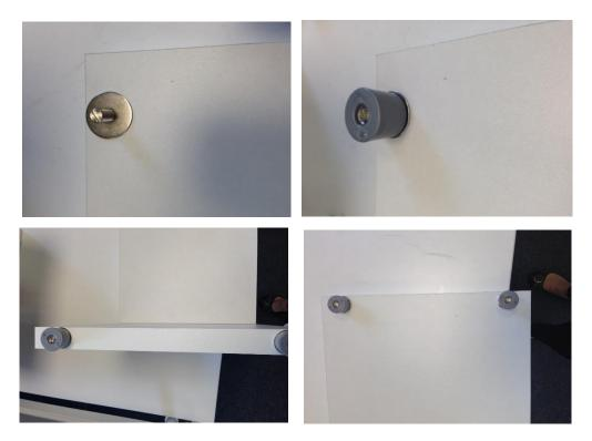
3. Starting at the bottom fix the panels together horizontally and vertically using the fixing kits.
